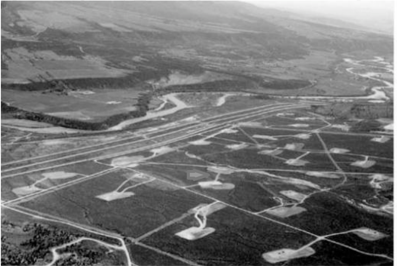
Aerial view of coalbed methane gas field in Colorado, USA
